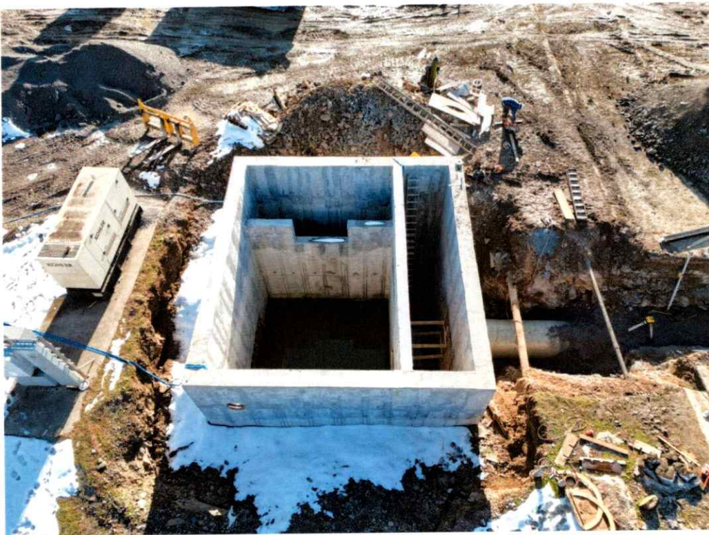
Pump Stations Construction Site
