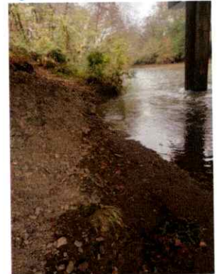
Sign Site 4 Removed
