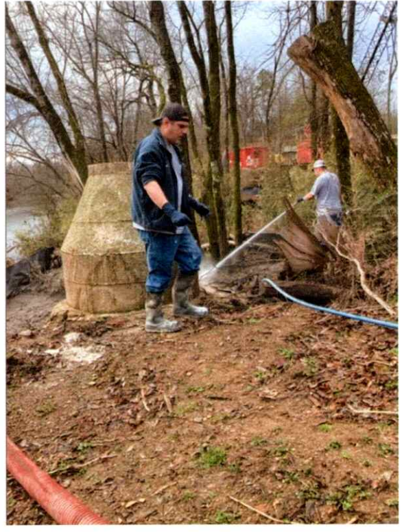
MH 1748 During Cleanup
