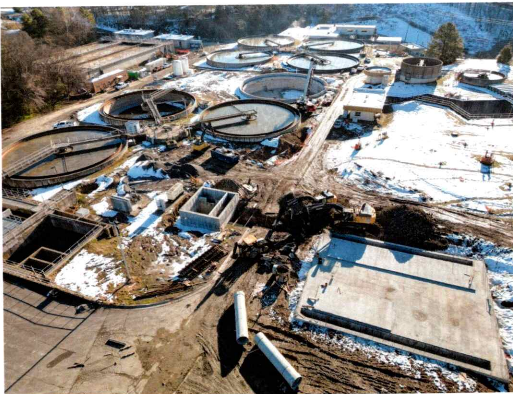
Clarifier Construction Site
