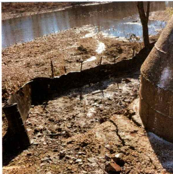
MH 1748 After Cleanup
