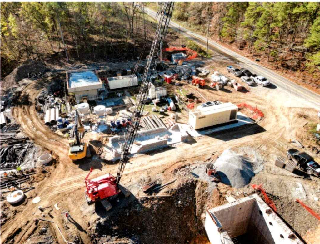
Pump Stations Construction Site
