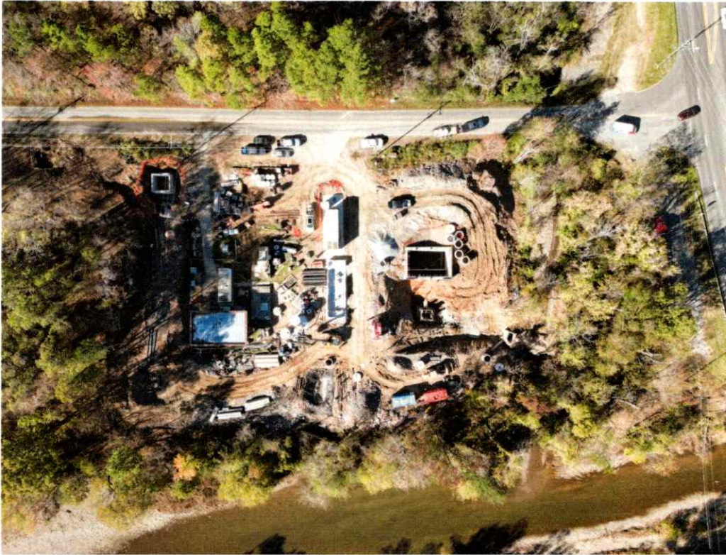
Pump Stations Construction Site
