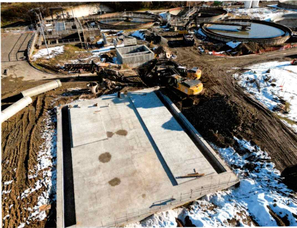
Clarifier Construction Site
