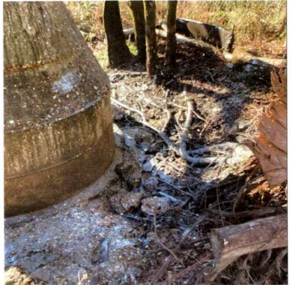
MH 1748 After Cleanup
