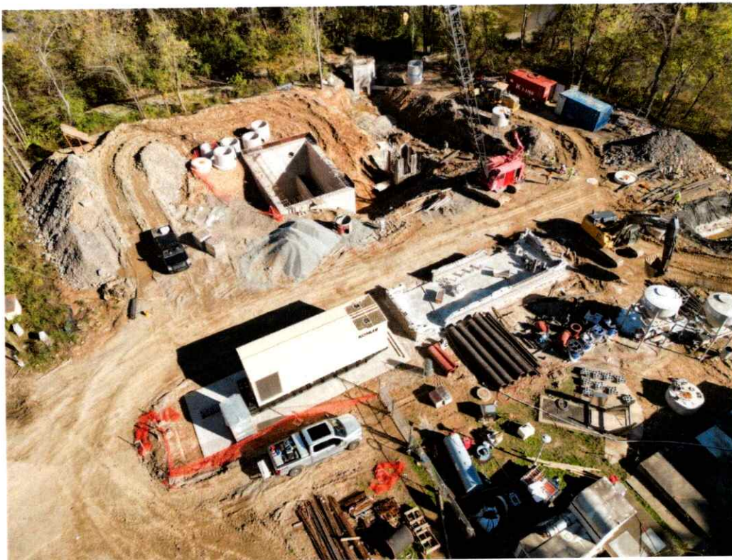
Pump Stations Construction Site
