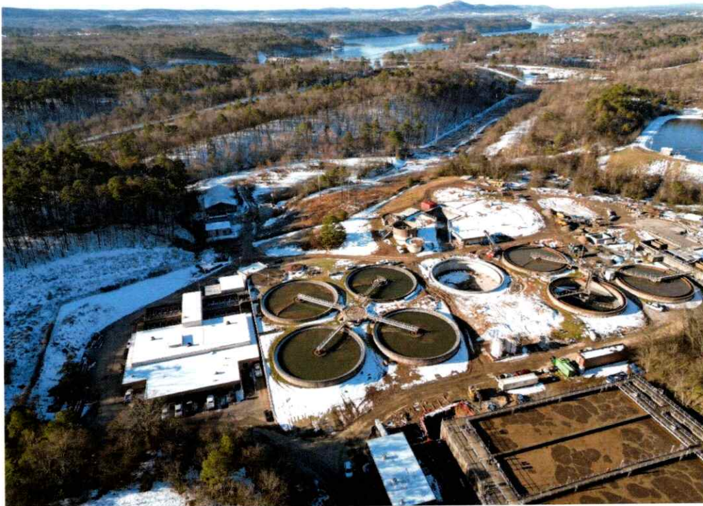
Clarifier Construction Site
