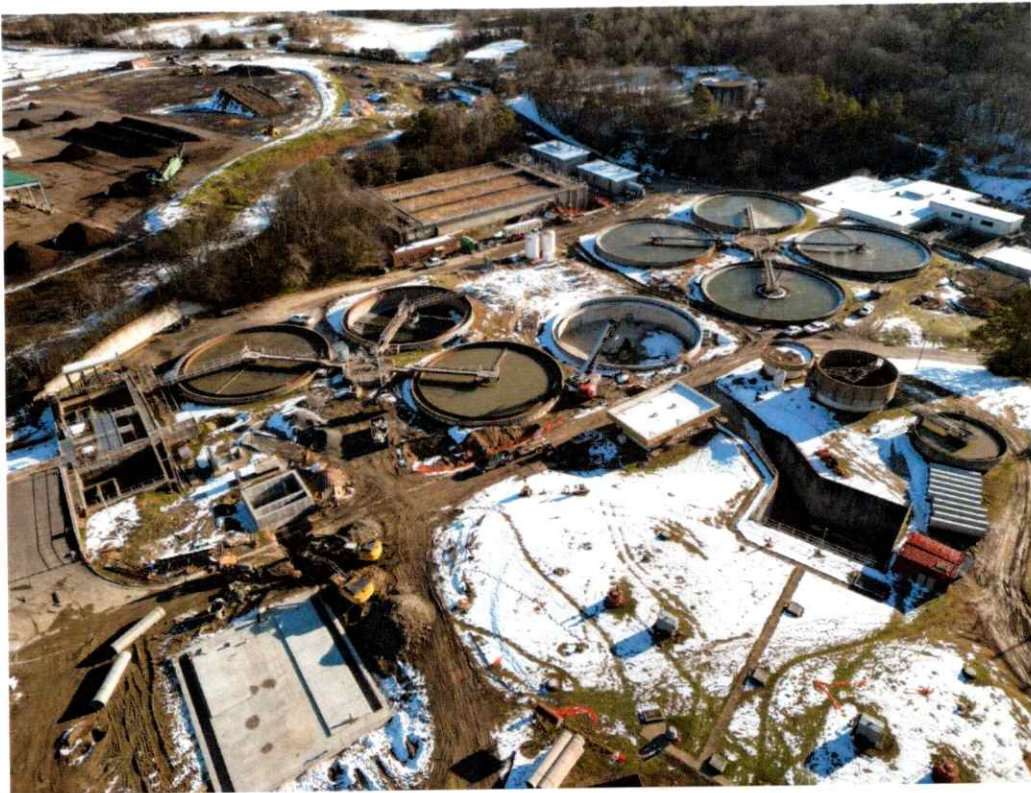
Clarifier Construction Site
