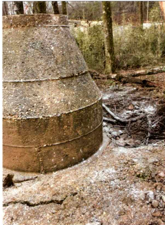
MH 1748 After Cleanup
